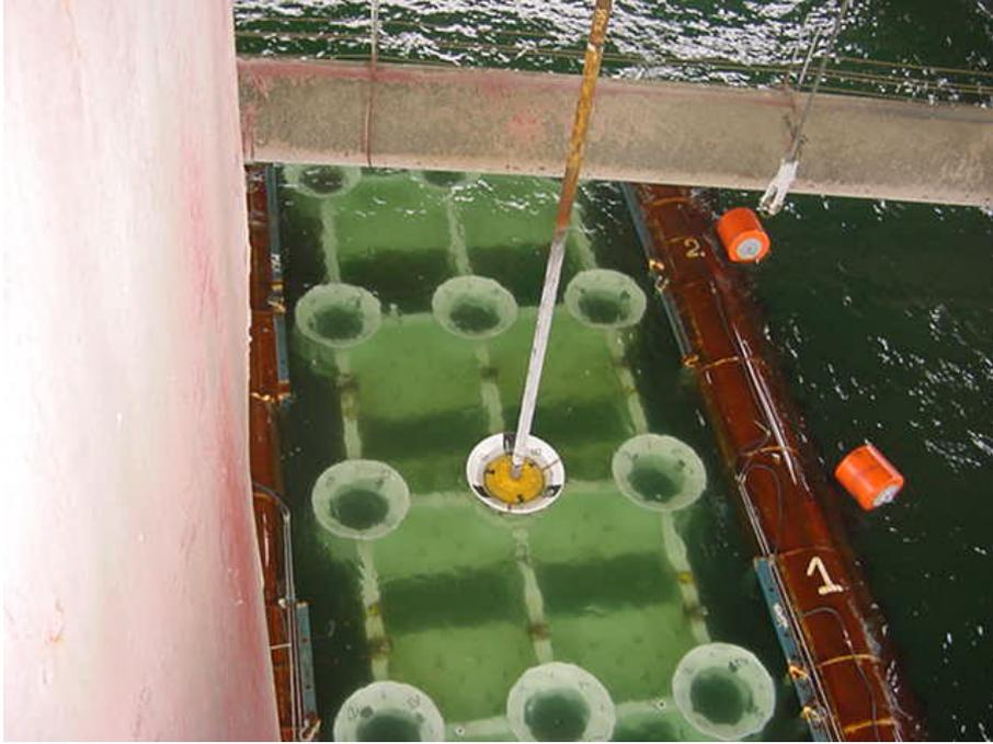
Figure 2: Drilling template being lowered into the sea using a riser
